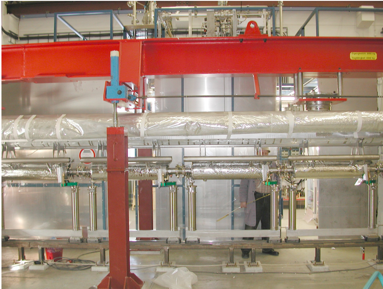
String in the assembly area Thomas Jefferson National Accelerator Facility
